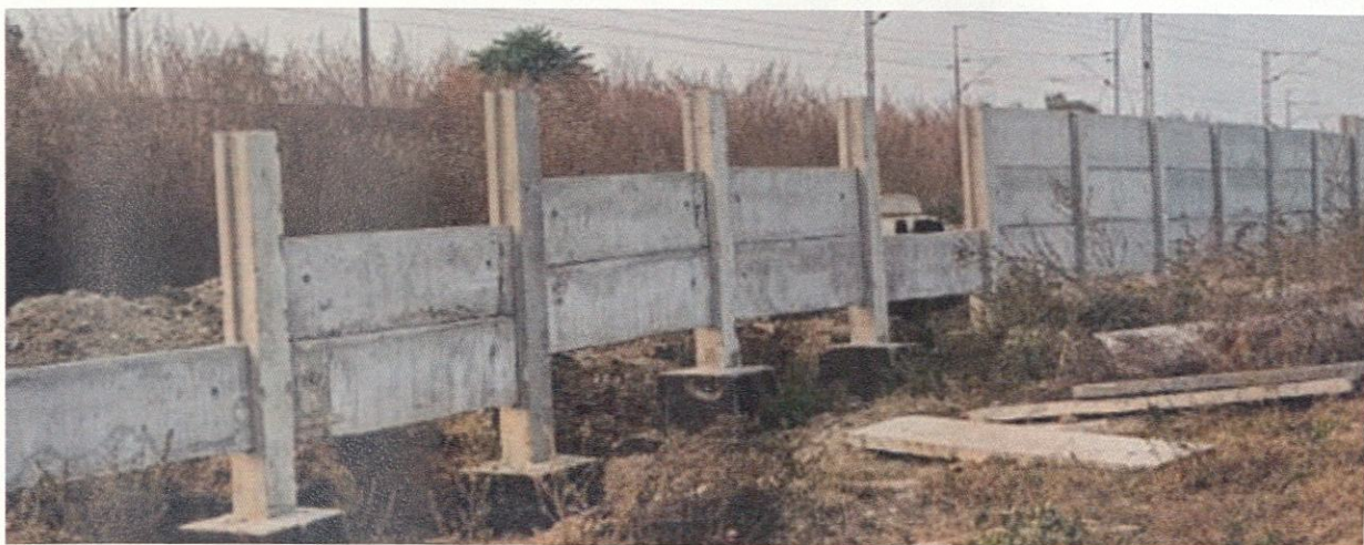
Figure 3.14.8: Concrete fencing under construction on the Nagpur-Butibori railway track segment.
