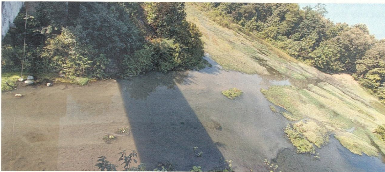
Figure 3.10.5: Water logging on both sides of the railway embankment on the Lalkuan-Chhatarpur railway track can make the drainage structures unusable by wildlife.
