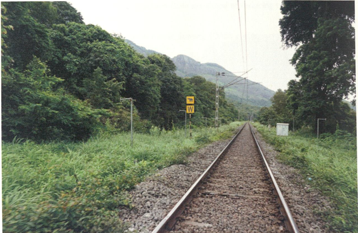
Signage (indicating elephant movement and with an instruction to whistle) and barriers along track B in the PGT-PDR section
