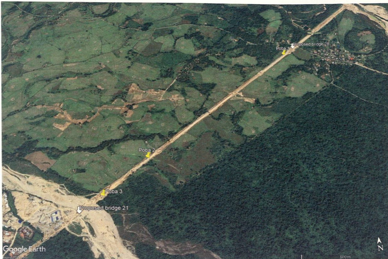
Figure 3.1.5: Proposed/under construction bridges (white arrows) on the Jonai-Pasighat railway line, and elephant crossing zones (yellow pins) as indicated by Forest Department personnel. Ramps and level crossings for elephant movement are to be constructed at each of the three crossing points.
