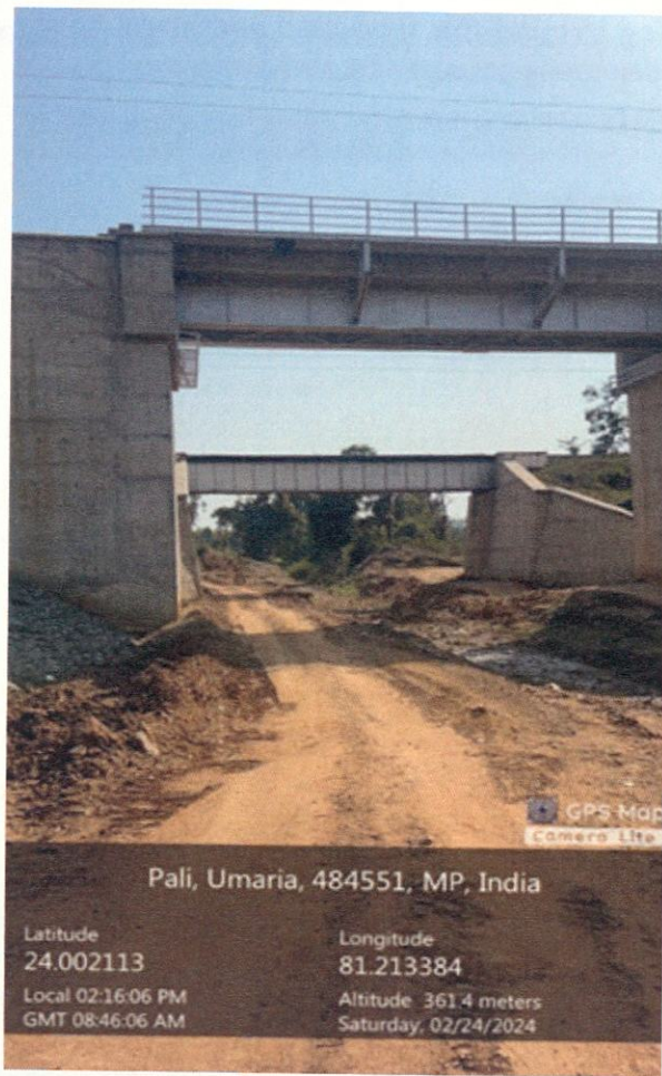
Figure 3.13.5: Underpasses being constructed on the Railway segment from Burhar to Shahdol Railway segment
