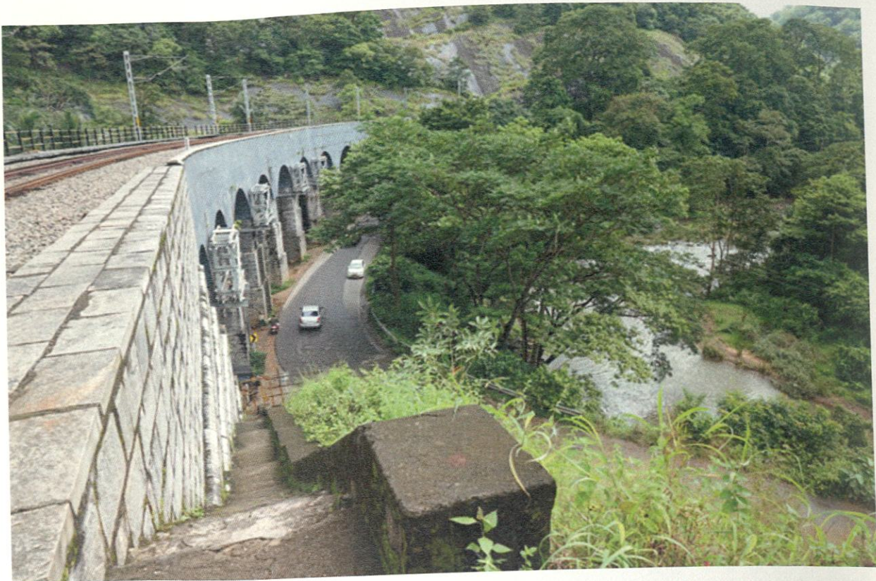
The Railway line is juxtaposed NH 744 in the entire stretch between Punalur and Tenkasi. Being mountainous, elephants cross the Railway line and the road only in a few locations
