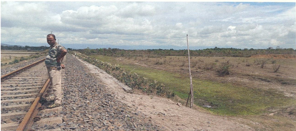
Figure 3.3.13: Low-voltage live-wire fencing used by villagers against crop-degradation by elephants along the Charduar-Bhalukpong railway line.
