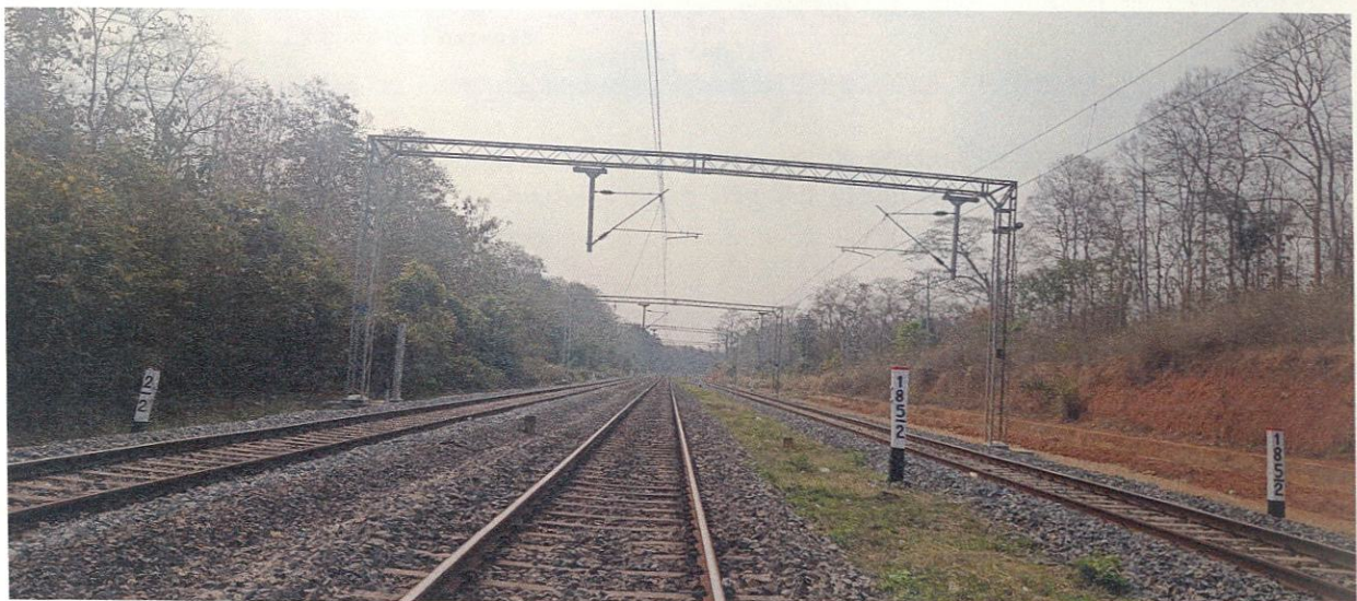
Figure 3.3.30: The space between parallel tracks should also be covered with the level crossing material recommended at elephant crossing sites.
