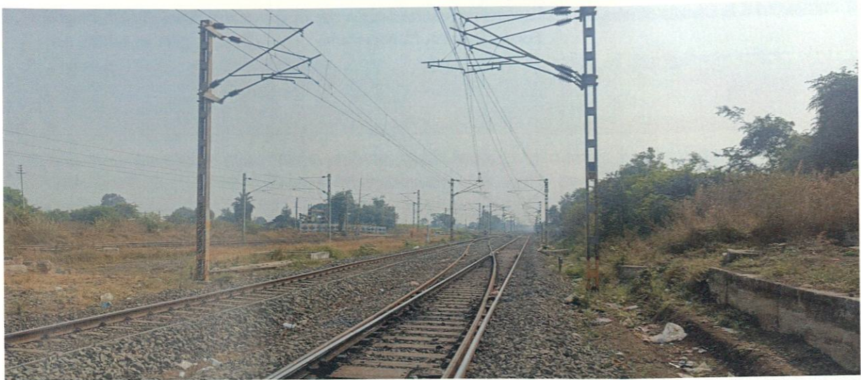
Figure 3.14.4: The Nagpur-Katol triple railway track in the Nagpur Forest Division.
