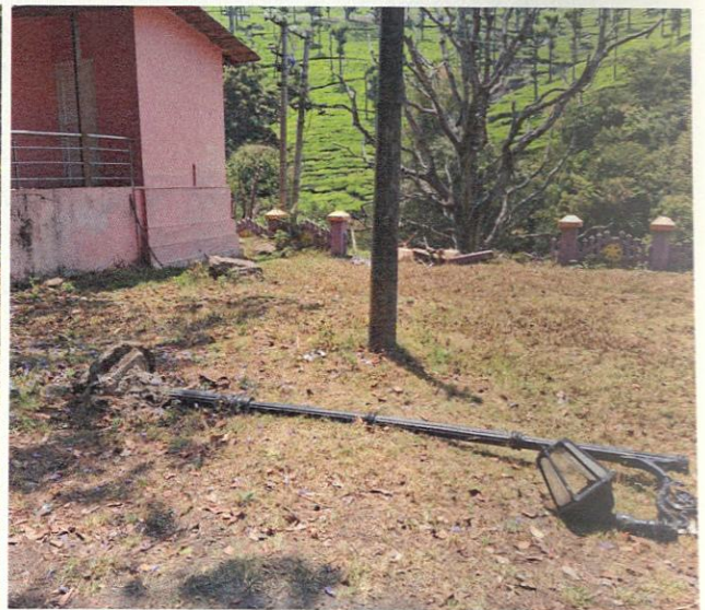
Figure 3.9.11: Damage by elephants at Runnymede station on the Kallar – Ooty railway line.
