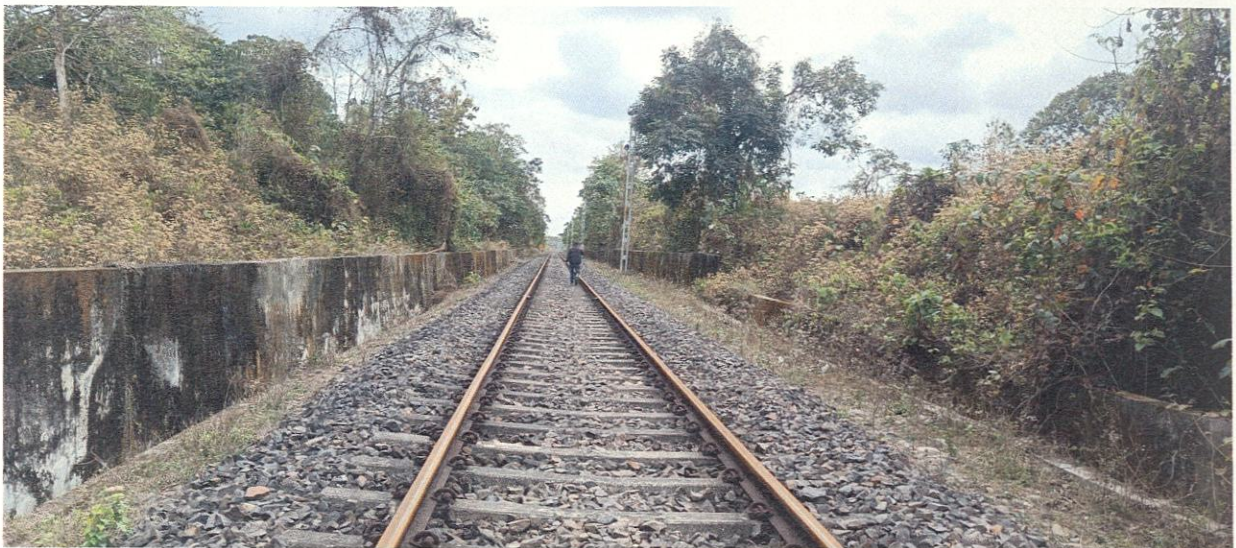
Figure 3.3.12: Concrete walls along two sections of the railway line Kalabil (Ch. 15/2 – 15/6), and that near Gamani Ban Gaon (Ch. 22/0 – 22/4) could cause elephants and other wild animals from getting stuck in the rail corridor. Multiple animal signs were found here.
