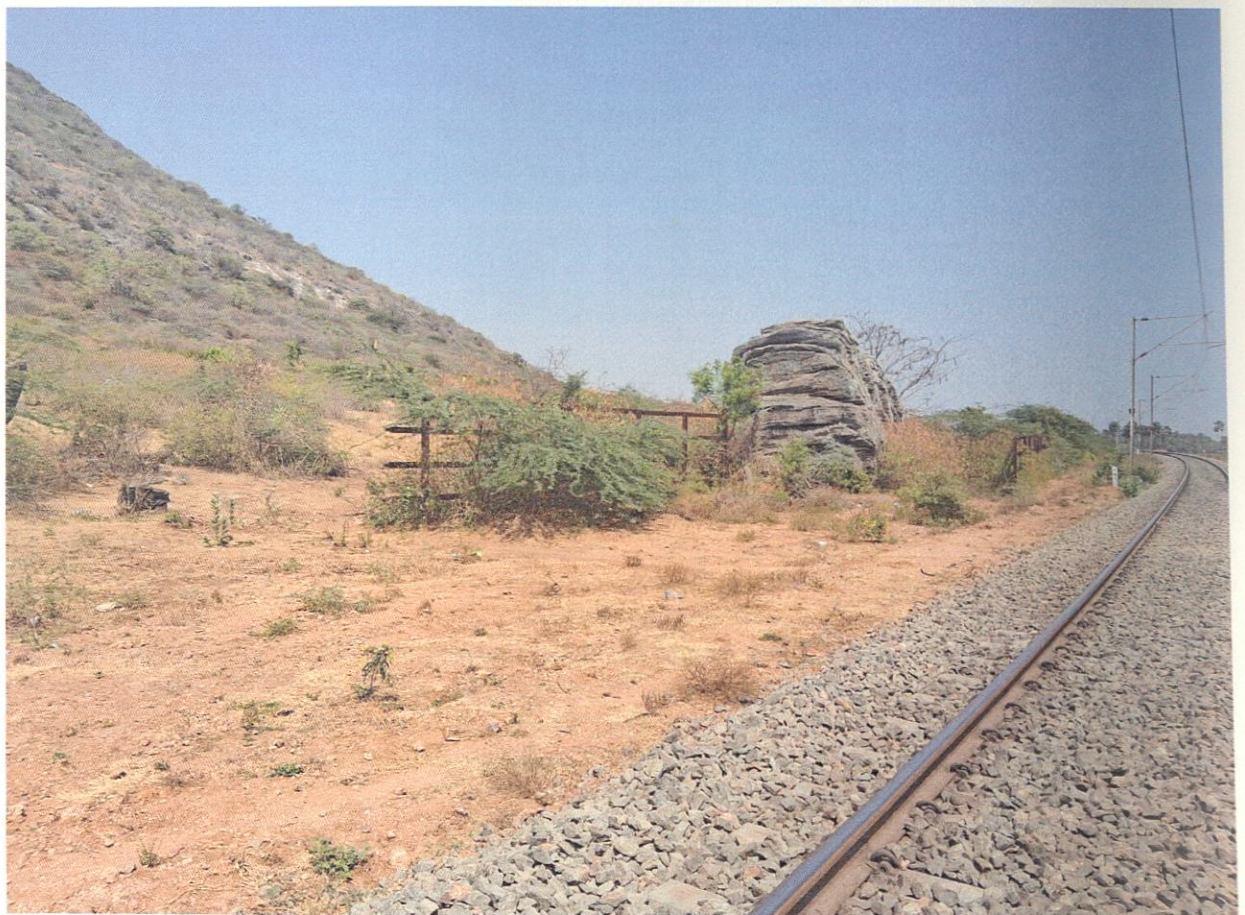
Figure 3.9.7: The old broken barriers along the Madukkarai – Ettimadai track used to stop elephants from walking on the track and crossing into the agricultural field (Chainage 498/9).
