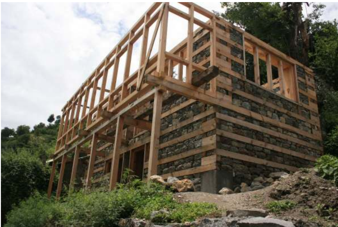
New house being constructed in traditional style
