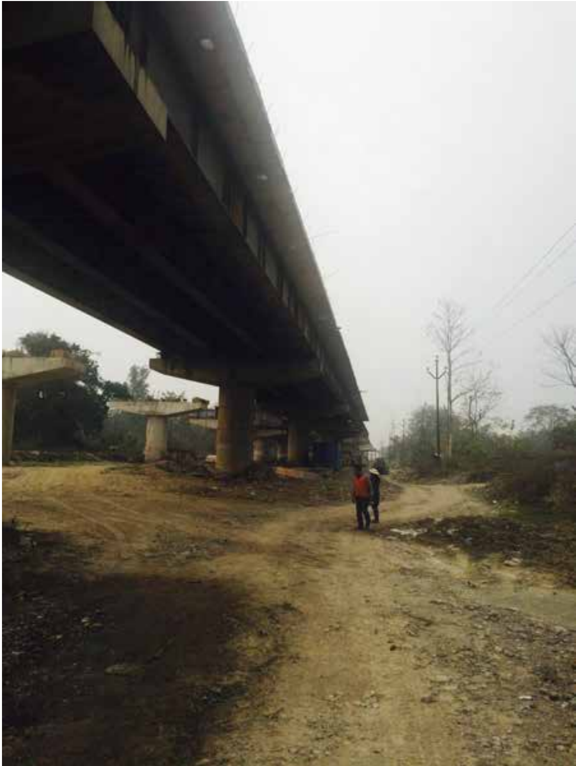
Figure 36: Under construction elephant crossing (736 m long) on NH – 72 (Rajaji National Park)
