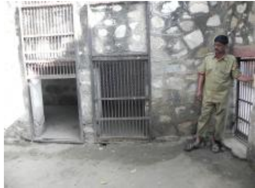
d. Concrete chamber for jackals inside the enclosure in Jaipur
