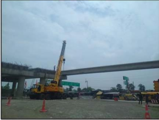
a. Construction activity
