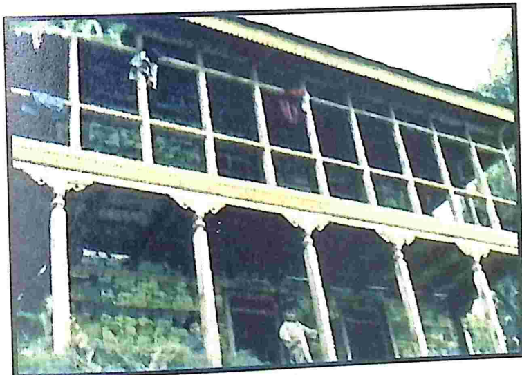
Timber Dependence for House Construction
