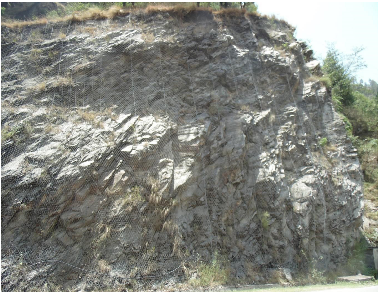
Landslide restoration along Badrinath Road, Nanda Devi Biosphere Reserve
