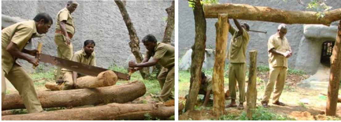
Plate 59: Log perches being constructed
