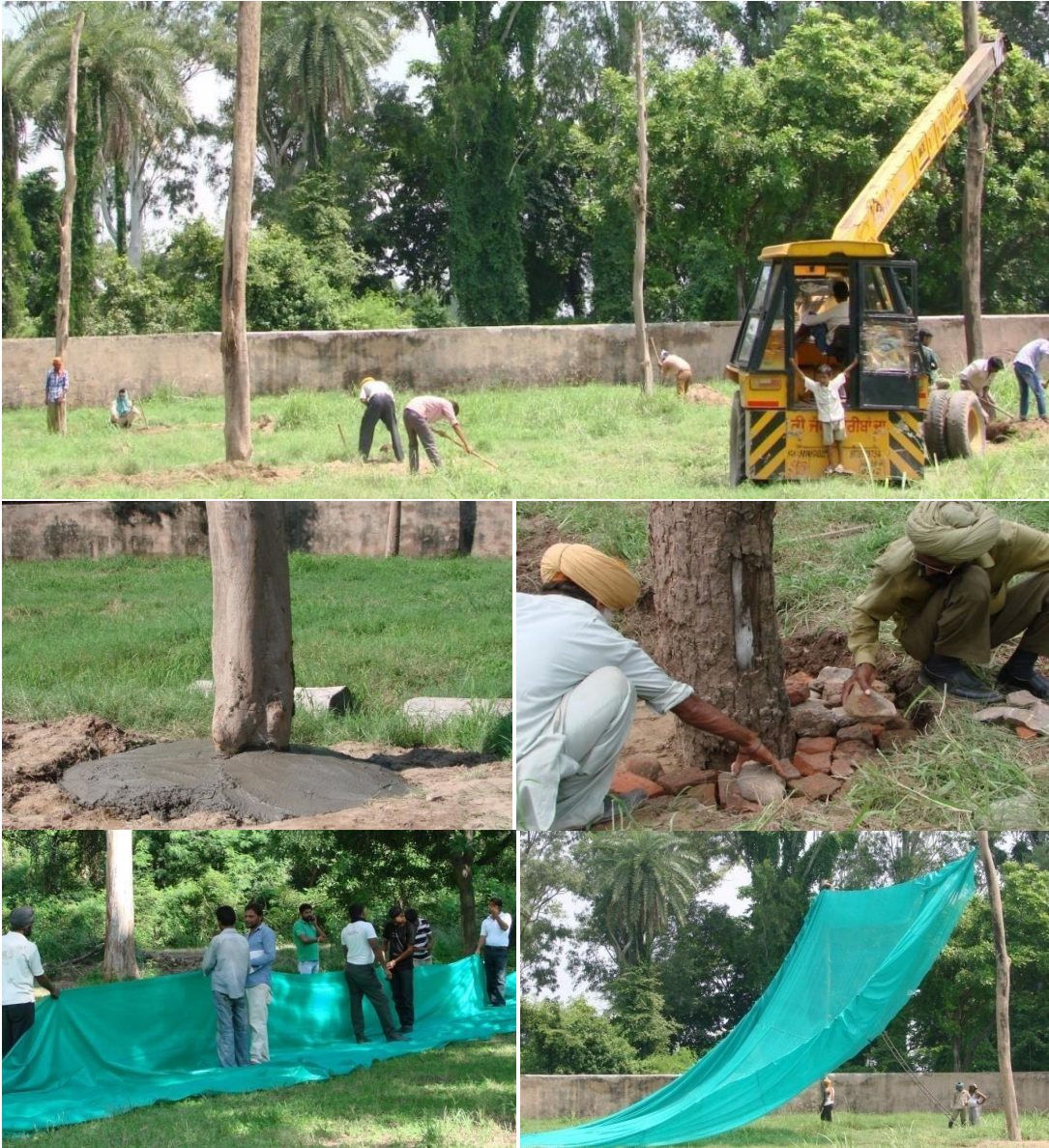
Plate 115: Step-wise set up procedure for temporary shed
