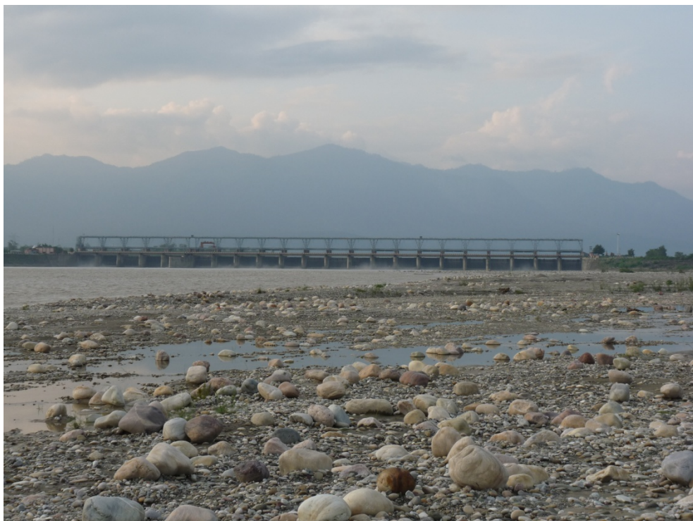
Plate 4.1 Barrage on Sharda River
