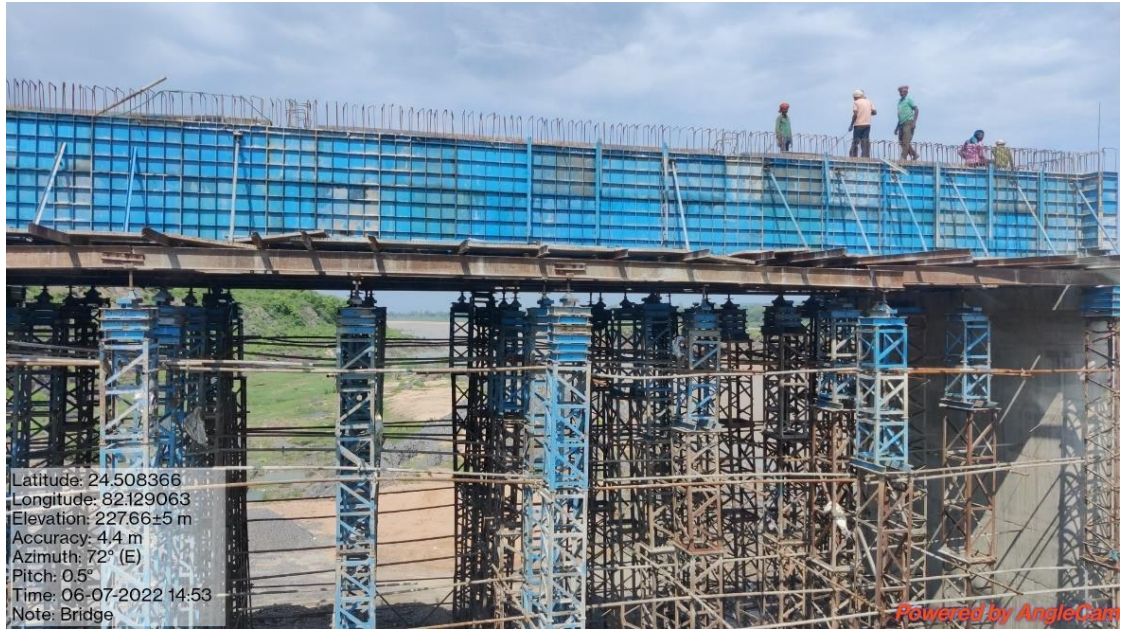
C. Construction work on the bridge being carried out
