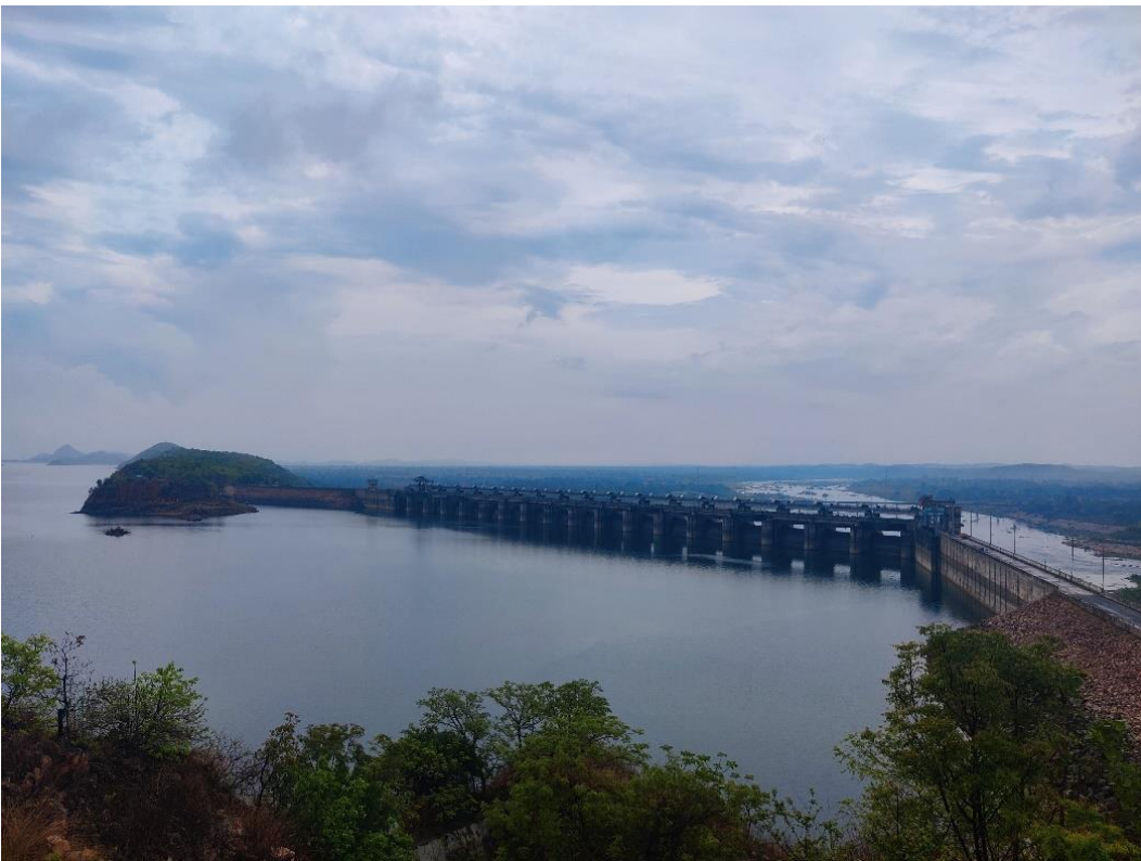
P. View of the Bansagar dam on the son River
