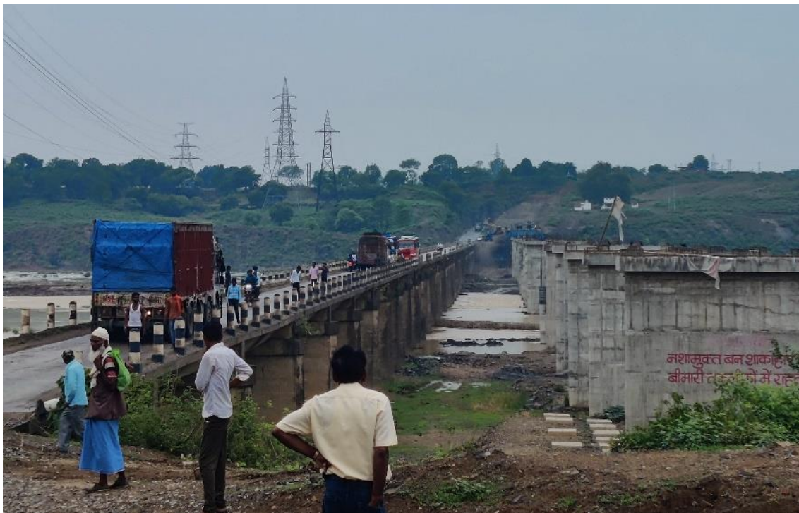
D. Traffic during vehicular movement in the old bridge
