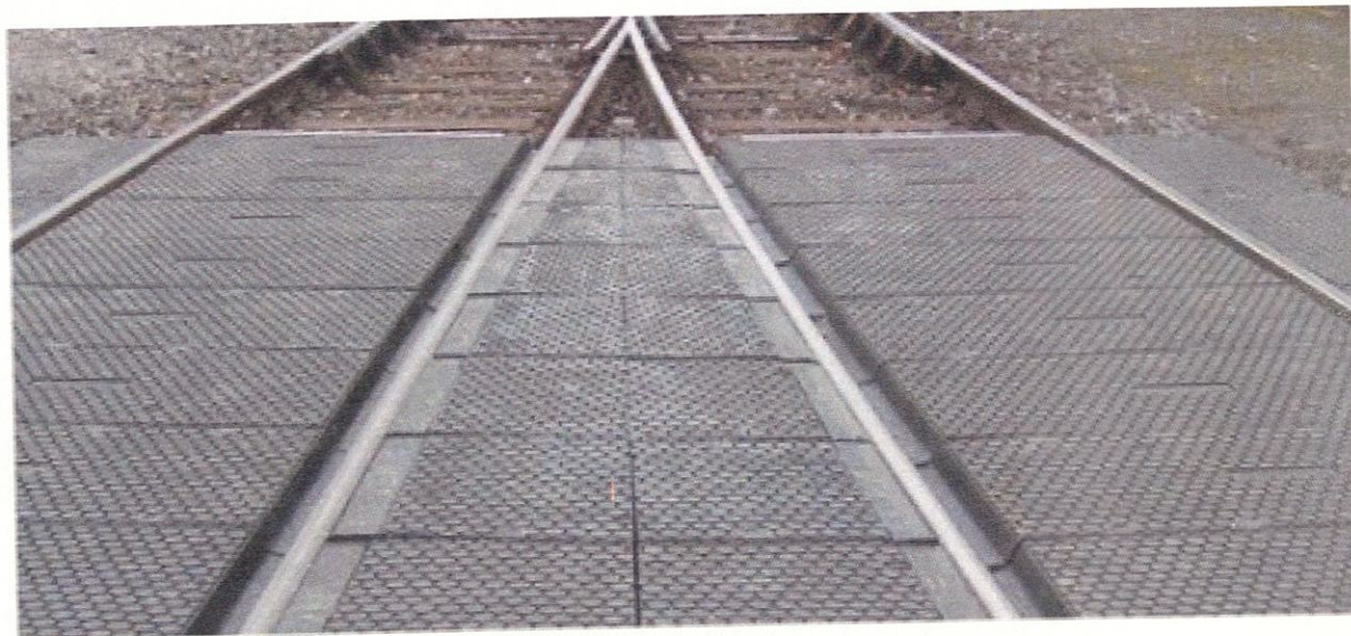
Figure 1. A level crossing with a rubberised surface that can be replicated on level crossings for wildlife.
