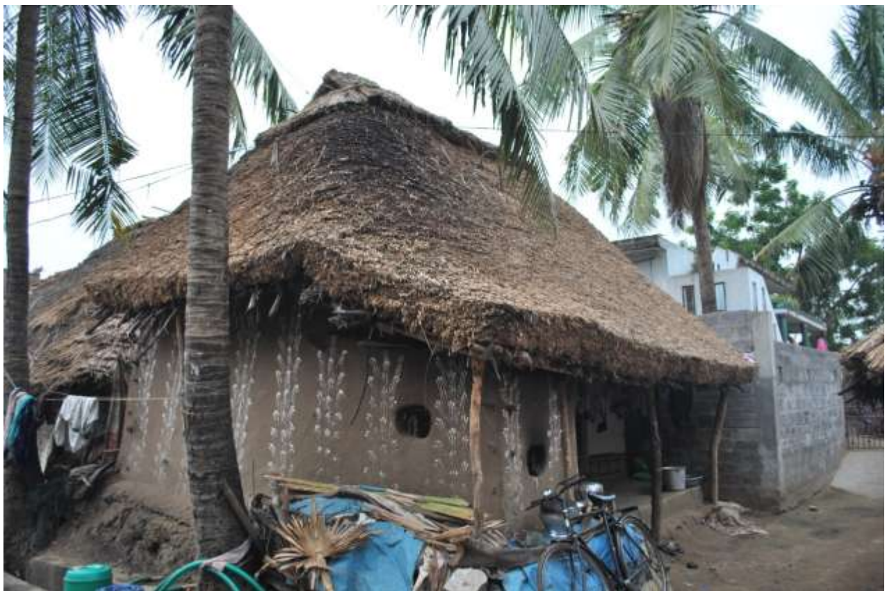
Figure 7: A typical ' kutcha ' house of local fishing community with roof covered by locally available grass species
