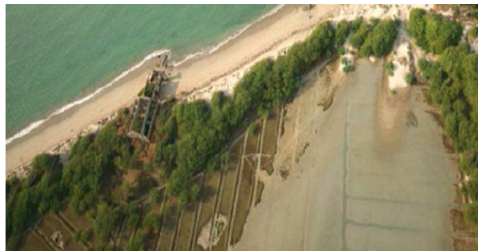
Parallel canal banking tried in Pamban
