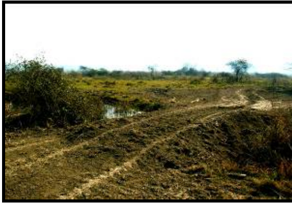
Plate 9.6 Gully plugging to maintain water level in central wetland Other management interventions
