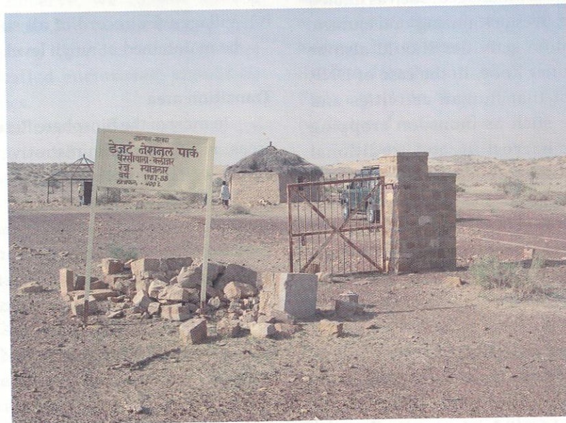
Fences should be repaired immediately
