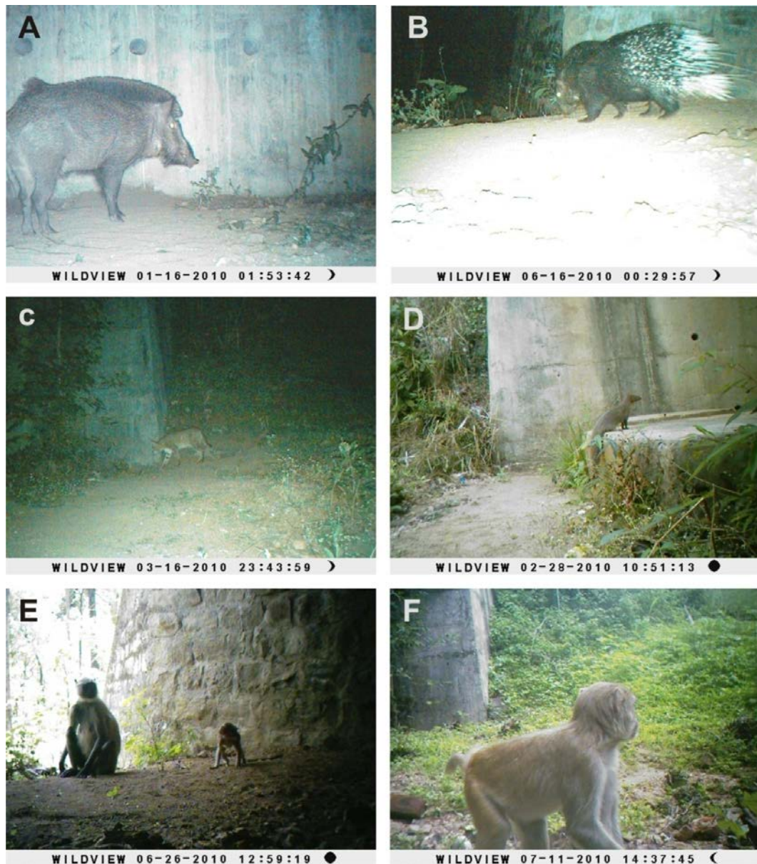
Figure 8.5 a Drainage culvert used by wild animals in Pench Tiger Reserve.
