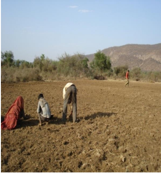
Plate 5.2. Clearing out vegetation manually for the site
