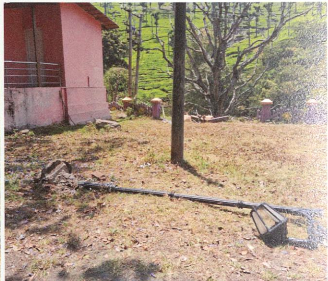
Figure 11: Damage by elephants at Runneymede station on the Kallar – Ooty railway line.
