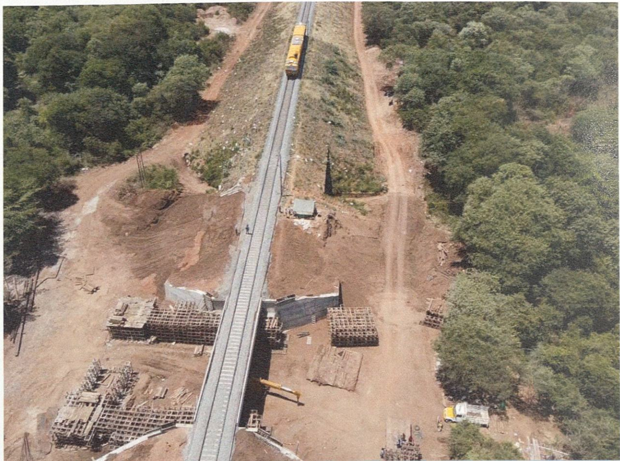
Photographs depicting the process of construction of elephant underpass on a railway line in Tamil Nadu
