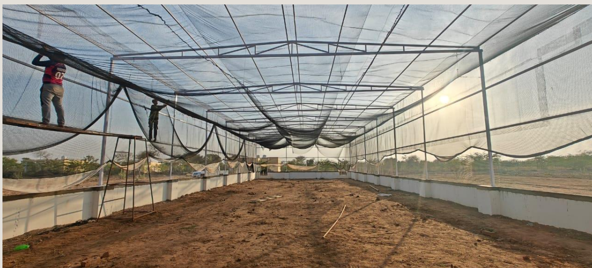
Image 36. Ongoing construction of Arwar LF Conservation Breeding Centre
