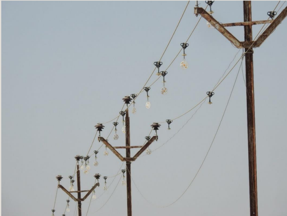
Image 34. Pilot installation of bird flight diverter in Mokla and Khetolai for mitigating power lines collision for Bustard conservation
