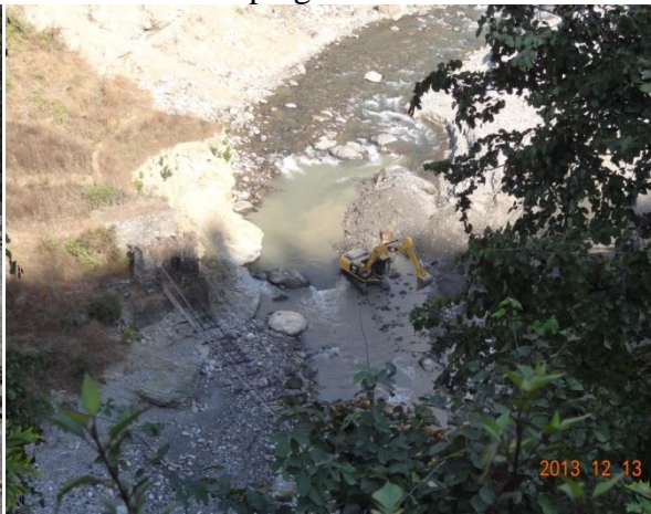
D-Removing sand for dam construction
