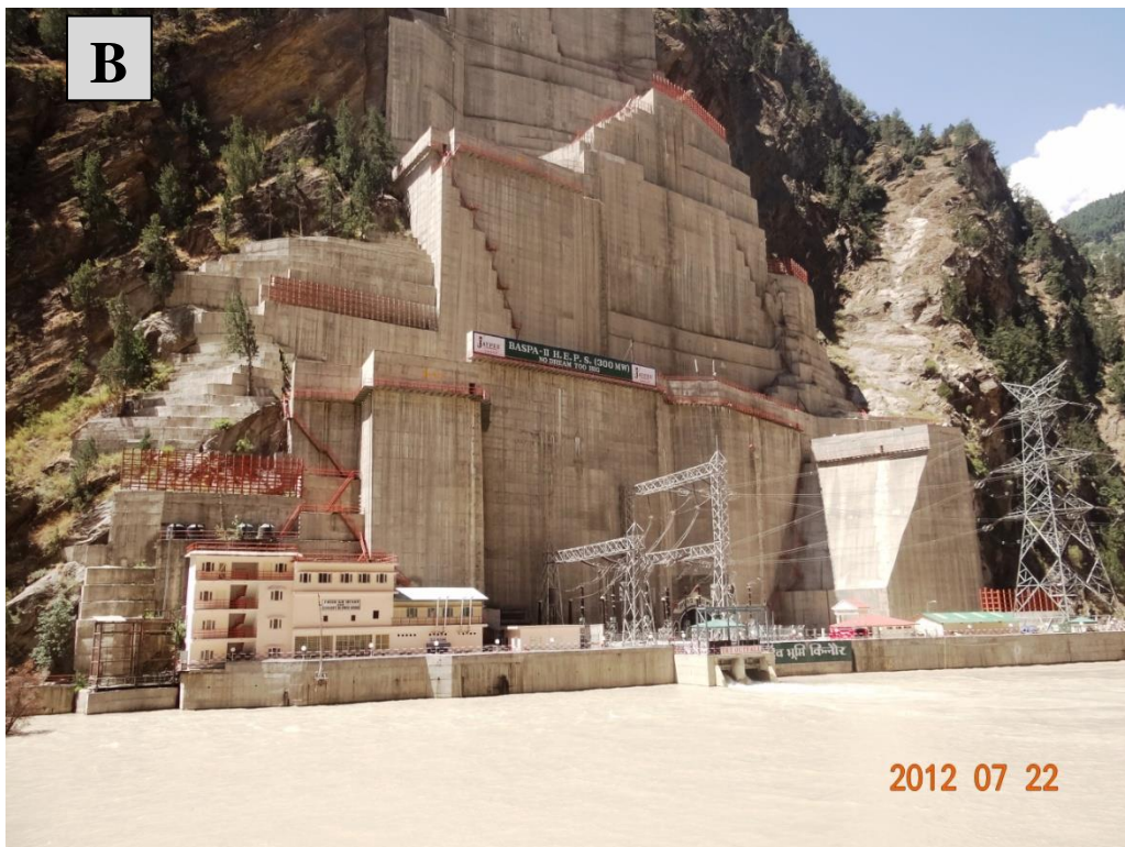
Plate 4. View of hydro power projects, Sutlej River: A-Constructing phase, B-Existing project
