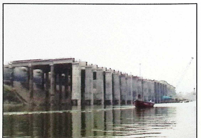
Construction of Jetty near Ramnagar
