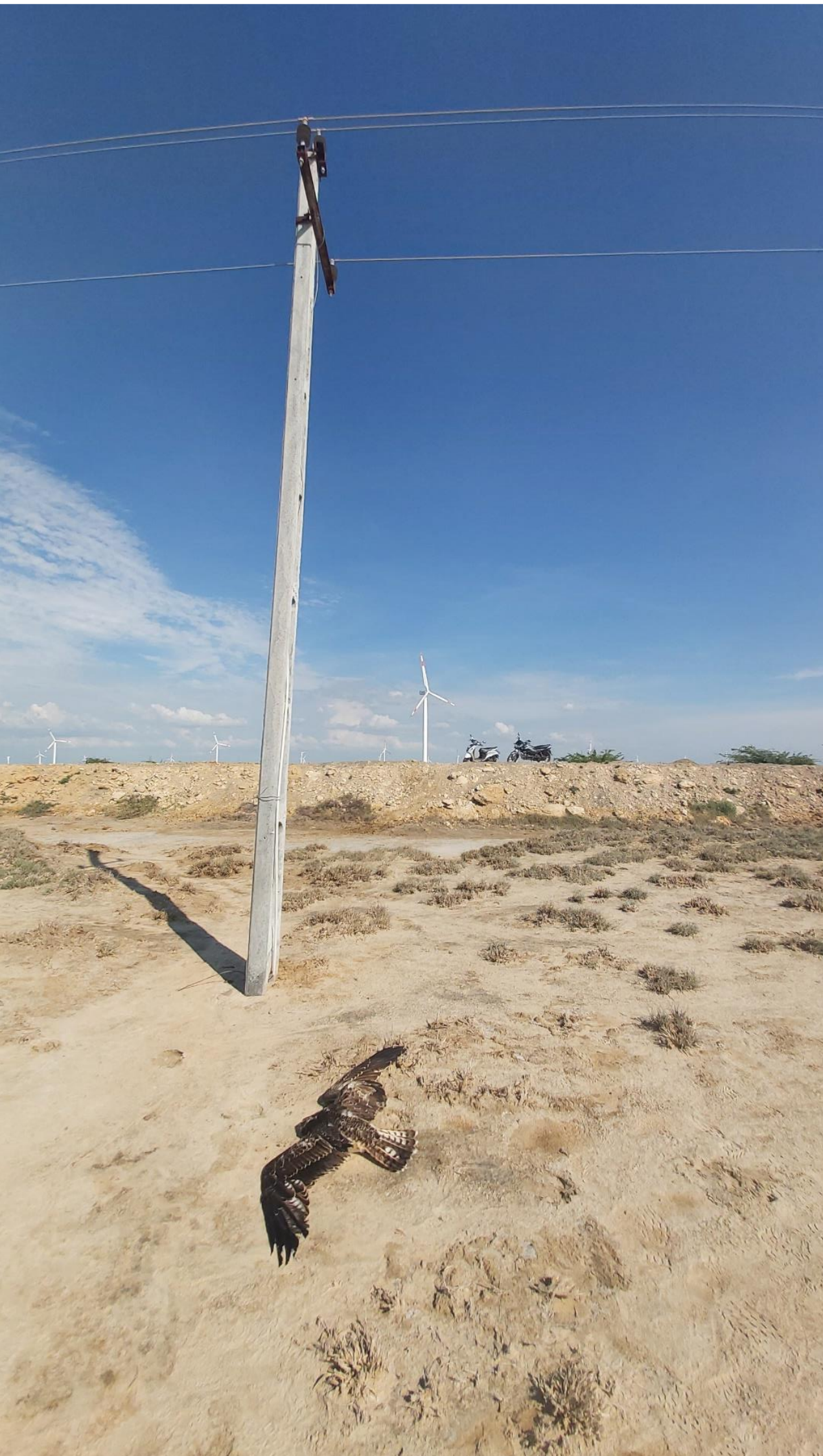
A carcass of an Osprey, lying under the distribution line. The burn of wing feathers suggested the electrocution mortality.
