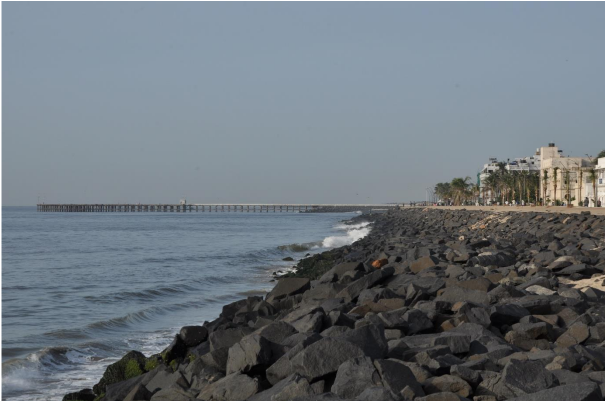
Figure 6 Beach armoring to protect coastal infrastructure along Puducherry coast
