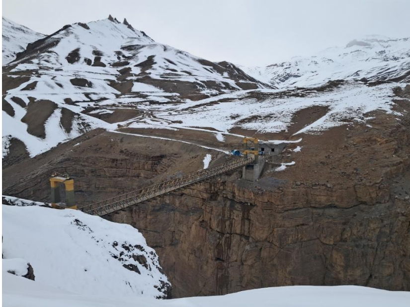
Plate 3: Chicham Bridge, Asia's highest suspension bridge at an altitude of 4037m (13,596 feet) connecting Kibber and Chicham villages in Spiti Valley (Source: Times of India).
