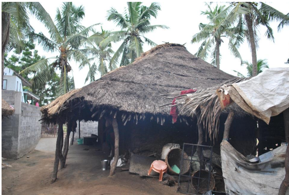
Figure 2.5. A traditional hut in a village adjoining the mangroves of Coringa Wildlife Sanctuary; Myriostachya wightiana , a mangrove associate species has been used as a thatching material for the roof.
