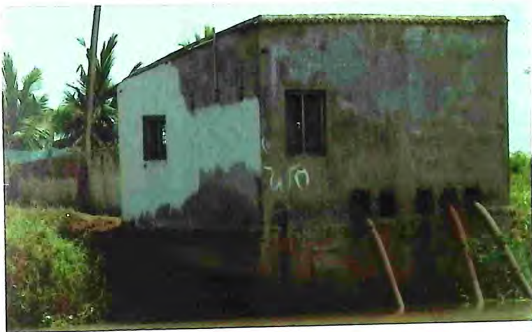
Plate 1 A Smooth coated otter holt below the pumping station of a Prawn culture pond near village.
