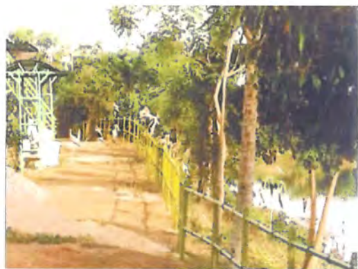
7d. Railing along the bund
