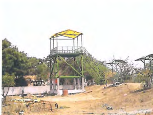
7e. Watch tower and sheds for visitors
