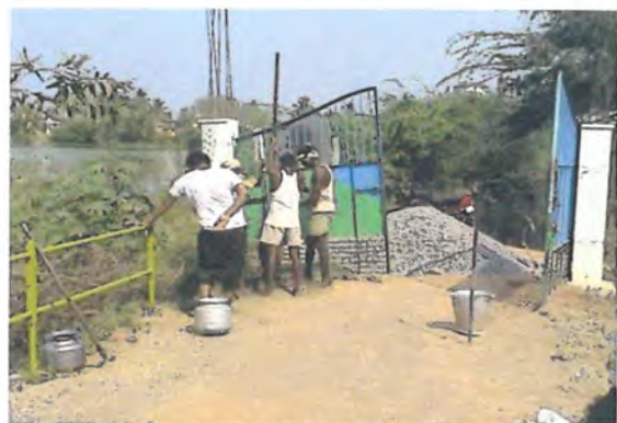
7f. Reconstruction of the entrance
