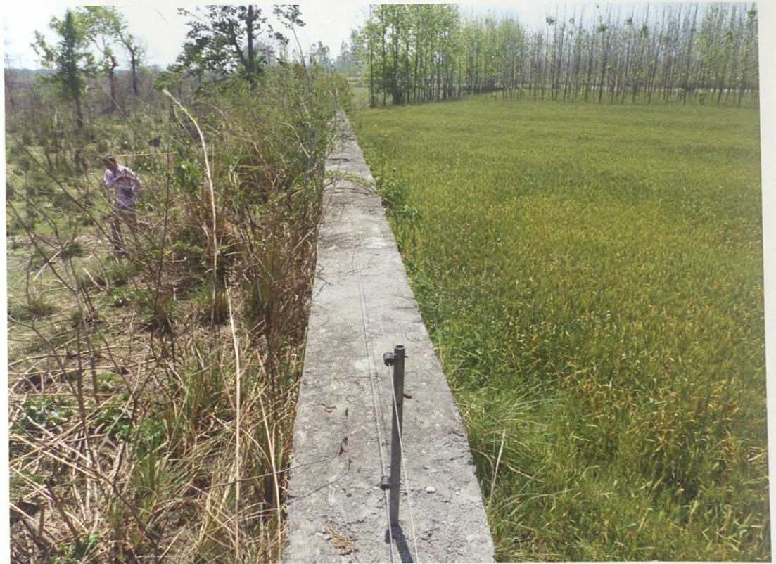
Composite barrier comprising of both wall and solar power fence
