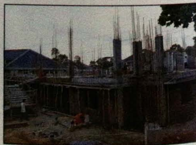
Construction of additional modular institutional block
