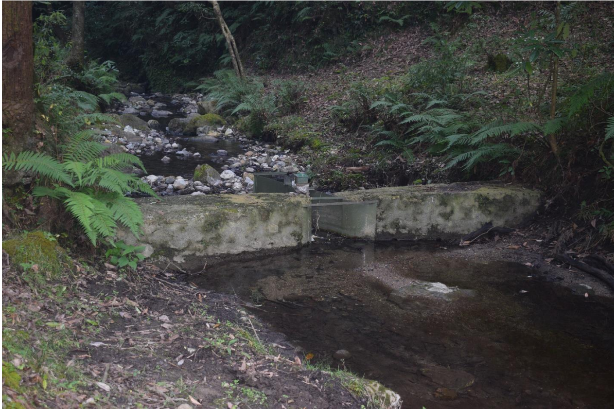
Photo 10: A check dam in stream of BWLS.
