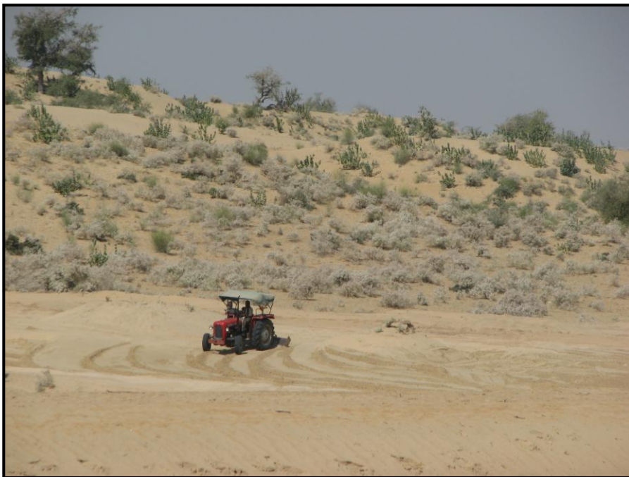
Plate 7.1 Clearing of vegetation for canal construction creates disturbance and changes in ecological character of the area.
