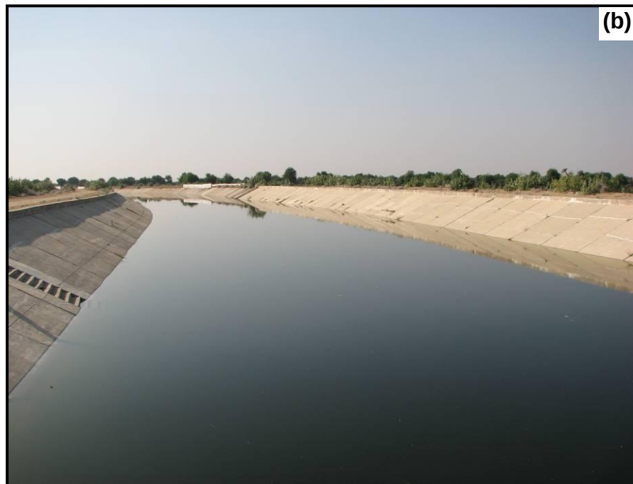
Plate 3.1 The Narmada Main Canal (NMC) of Rajasthan taking off from the tail of NMC of Gujarat near village Shilu of Sanchor tehsil of Jalor district(a) and the already constructed section of main Narmada Canal(b).
