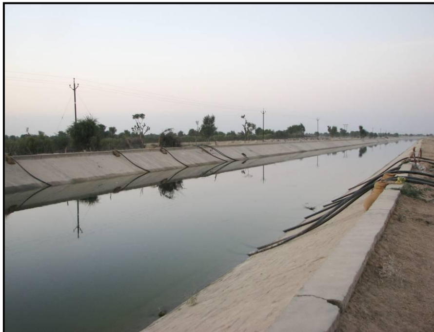
Plate 3.2 The canal is already becoming a source of water for local people.
