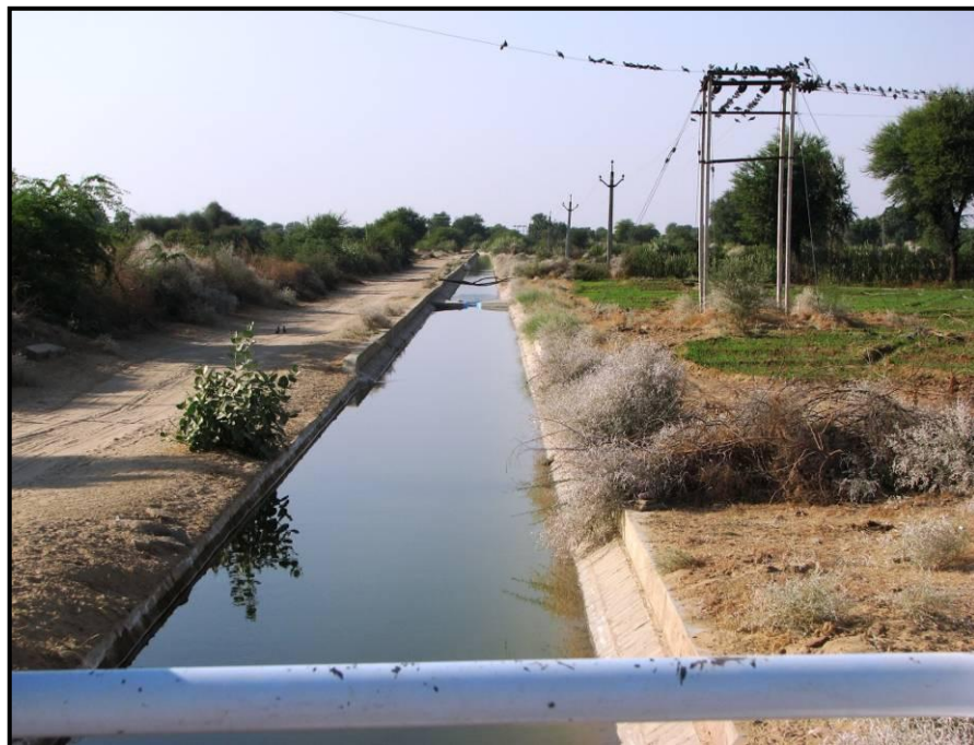
Plate 3.4 A typical lift and distribution system for serving the lift command area of the project.
