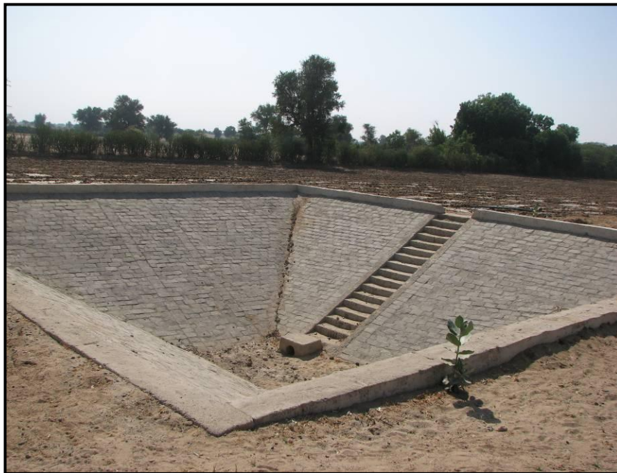
Plate 3.5 Pump house (a) A typical diggi that draws water from the minor canal from where the cultivators draw water through pumping system (b)
