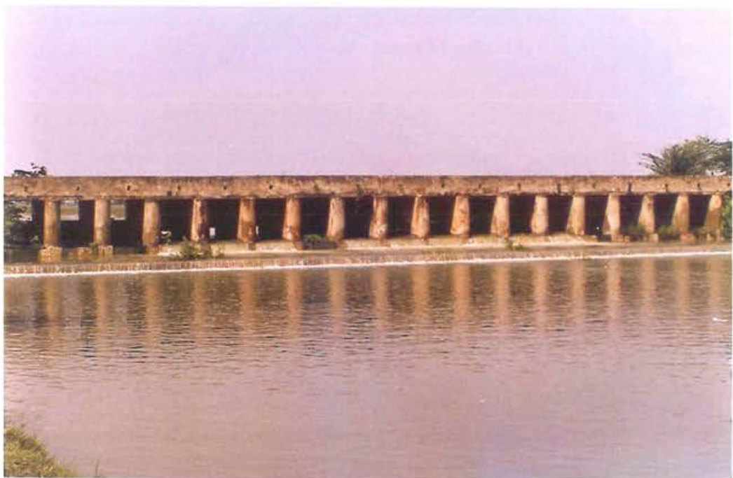
Plate 9. The Ajan Dam releases water to KNP through the sluice gates
