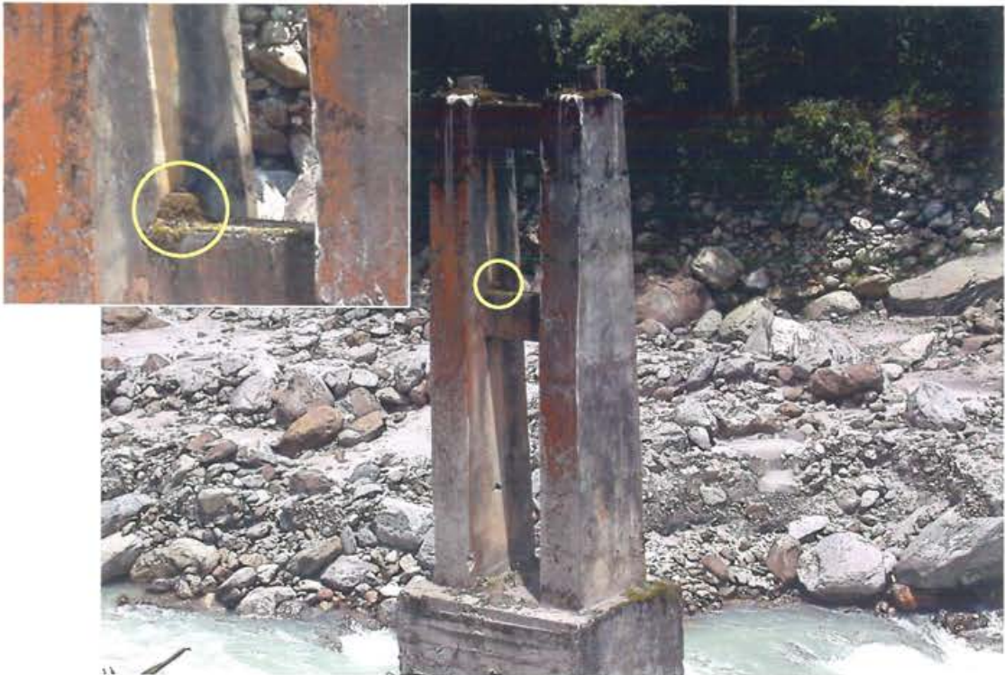
Plate 4.3 The nest of Blue Whistling Thrush placed in the pole of a bridge, enlarged view is shown in the inset. They build nests on rocky ledges or man made structures near the stream.
