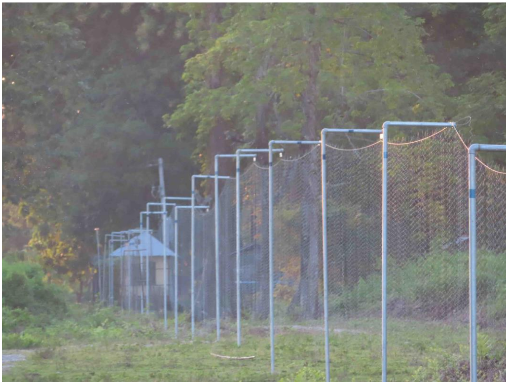
Figure 20: Hanging solar fences are a novel concept in human-elephant conflict management having recently been used in Sri Lanka, southern and north-eastern India with promising results; these fences are much higher than conventional fences (14 ft) and are also electrically charged (solar) to give a mild shock to elephants, who learn and adapt to avoid the fences and such areas; these fences hang like a curtain with a gap underneath for smaller animals to cross and cannot be toppled easily by force (Image courtesy Wildlife Trust of India, see https://youtu.be/FFhXWSaBPJA )
