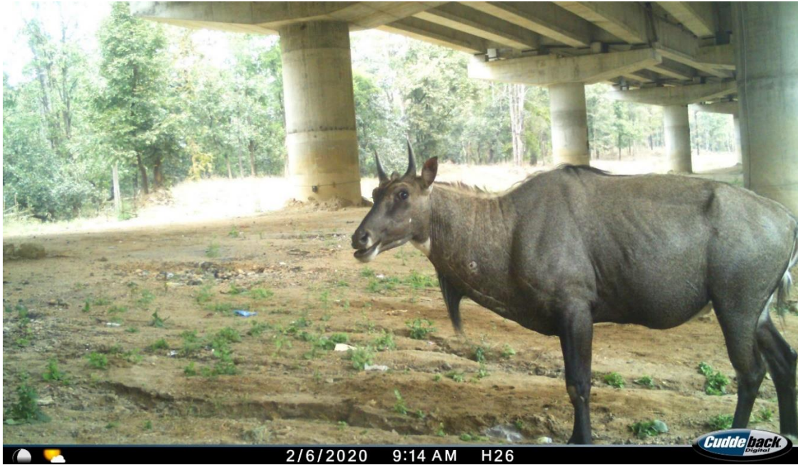
Figure 2.17. A nilgai or bluebull using one of the 9 wildlife crossing structures on National Highway 44 passing through the Pench Tiger Reserve, Maharashtra.
