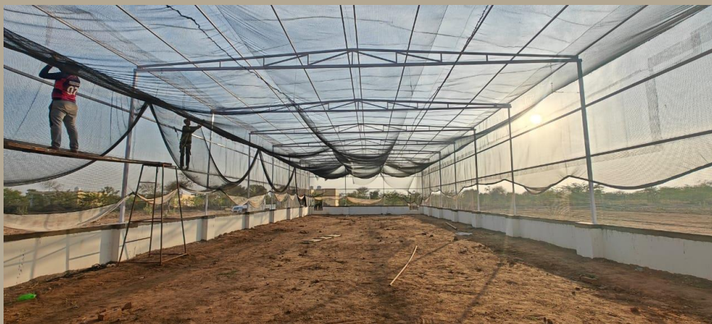
Image 22: Ongoing construction of Arwar LF Conservation Breeding Centre
