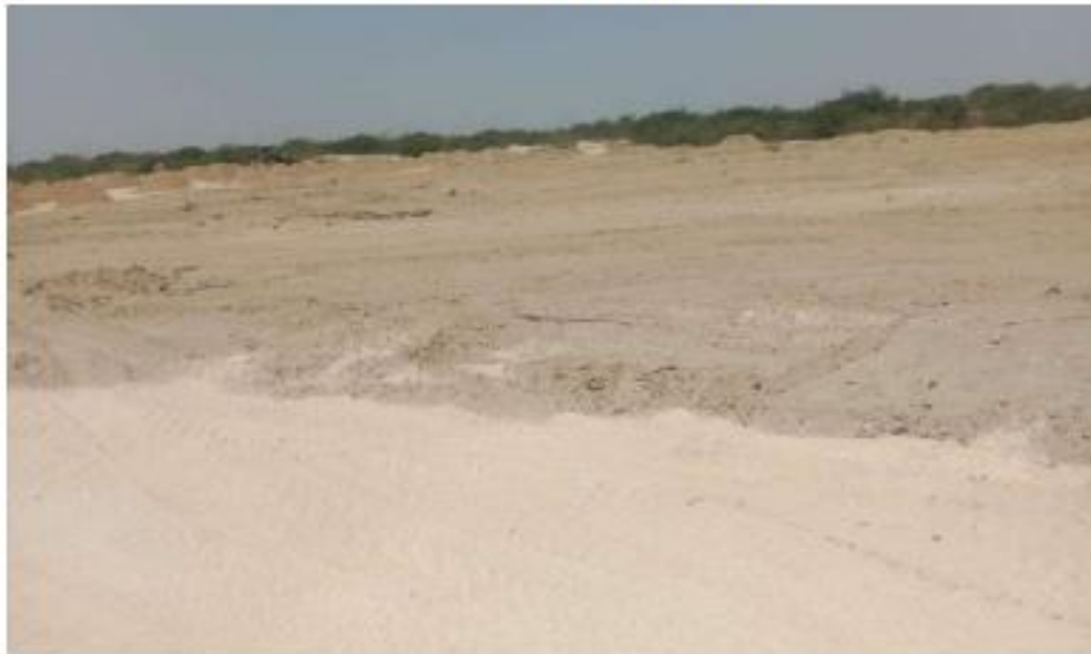
Mined out Levelled area at Sanu-II mines ( 1 st week of Sept'25)
