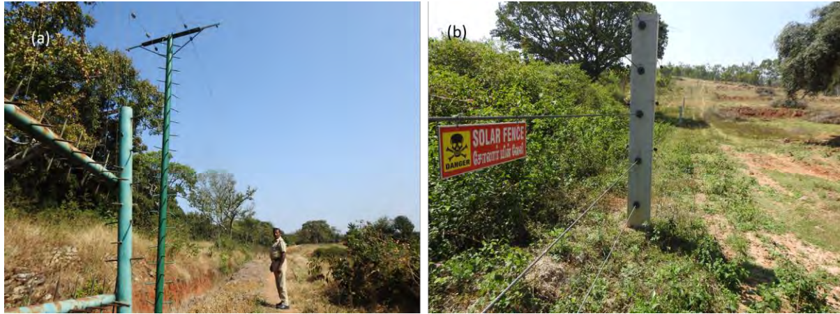
Figure 4.4 Mitigation measures deployed by the Forest Department to mitigate human-elephant conflict: (a) combination of elephant-proof trench, hanging solar fence and spike pillar fence (b) solar fence.
